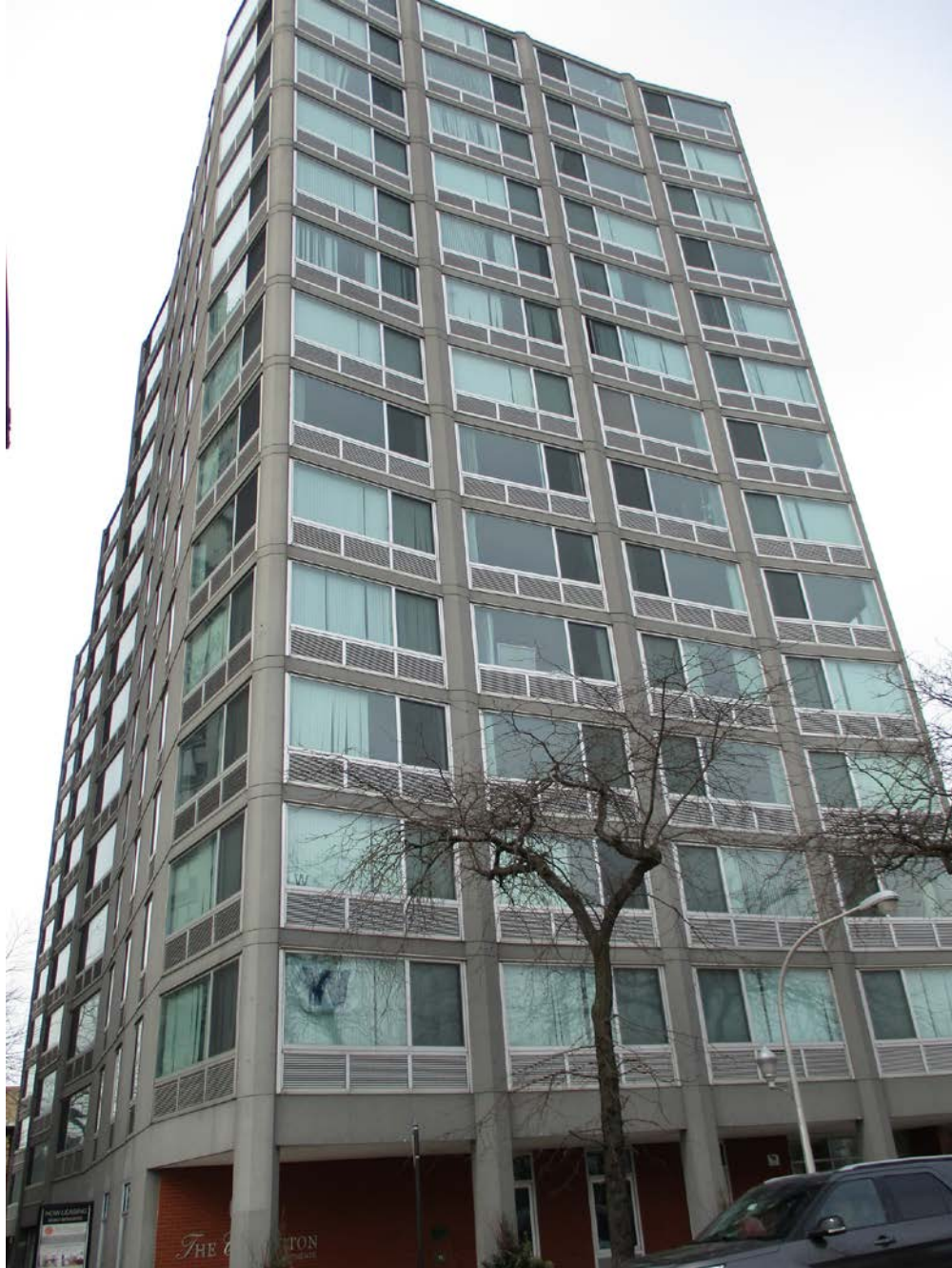
4600 N. Clarendon Avenue, view looking northwest from N. Clarendon Avenue toward East façade
