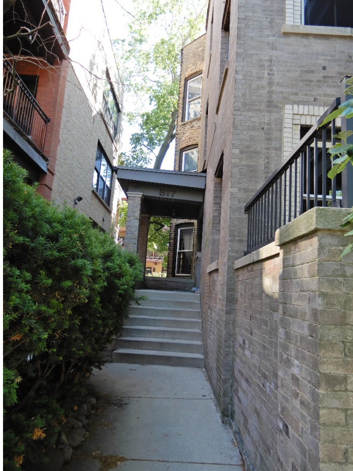
817 W. Lawrence Avenue, view looking south from W. Lawrence Avenue toward entryway
