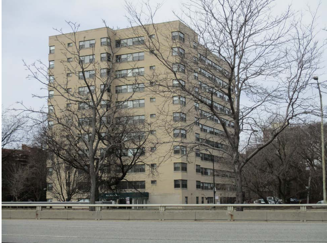
4200 N. Marine Drive, view looking southwest from N. Lake Shore Drive toward East and North façades
