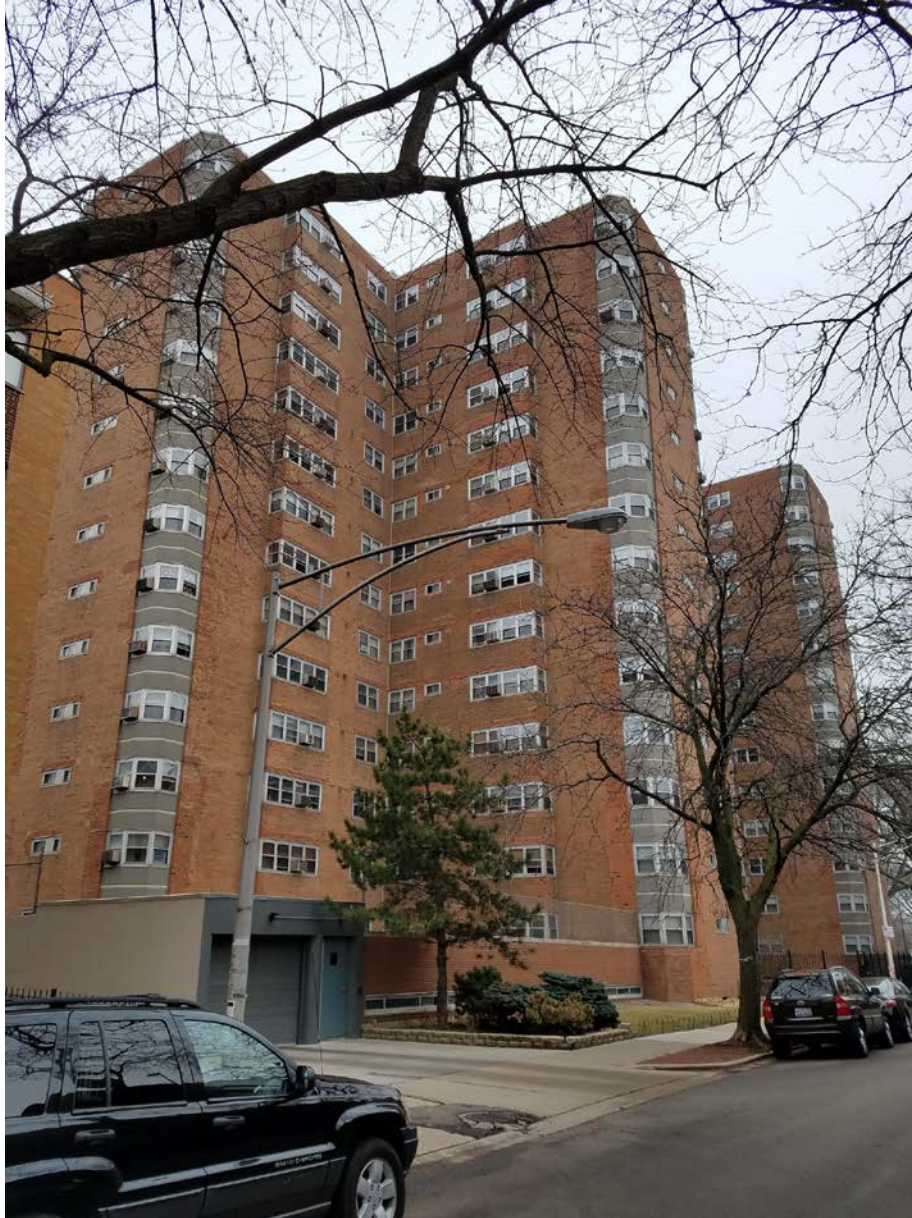
4950-4980 N. Marine Drive, view looking northeast from W. Margate Terrace toward South façade
