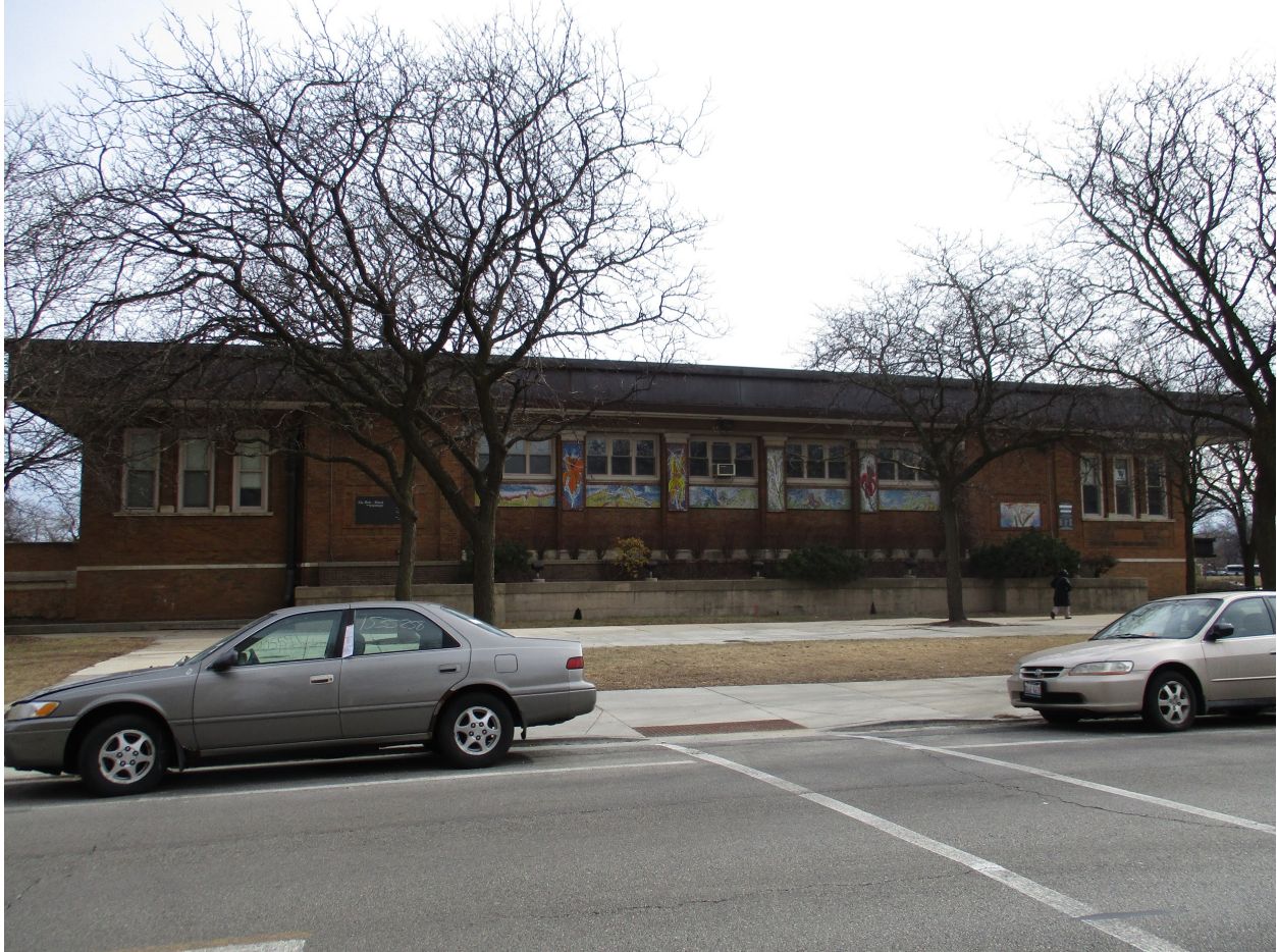
4501 N. Clarendon Avenue, view looking east from N. Clarendon Avenue toward West façade
