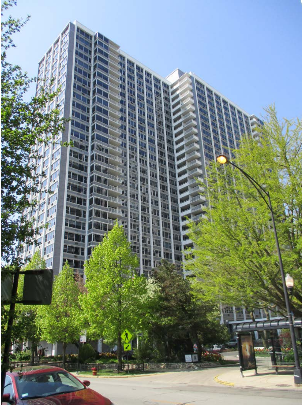
4250 N. Marine Drive, view looking southwest from N. Marine Drive toward North façade of South tower
