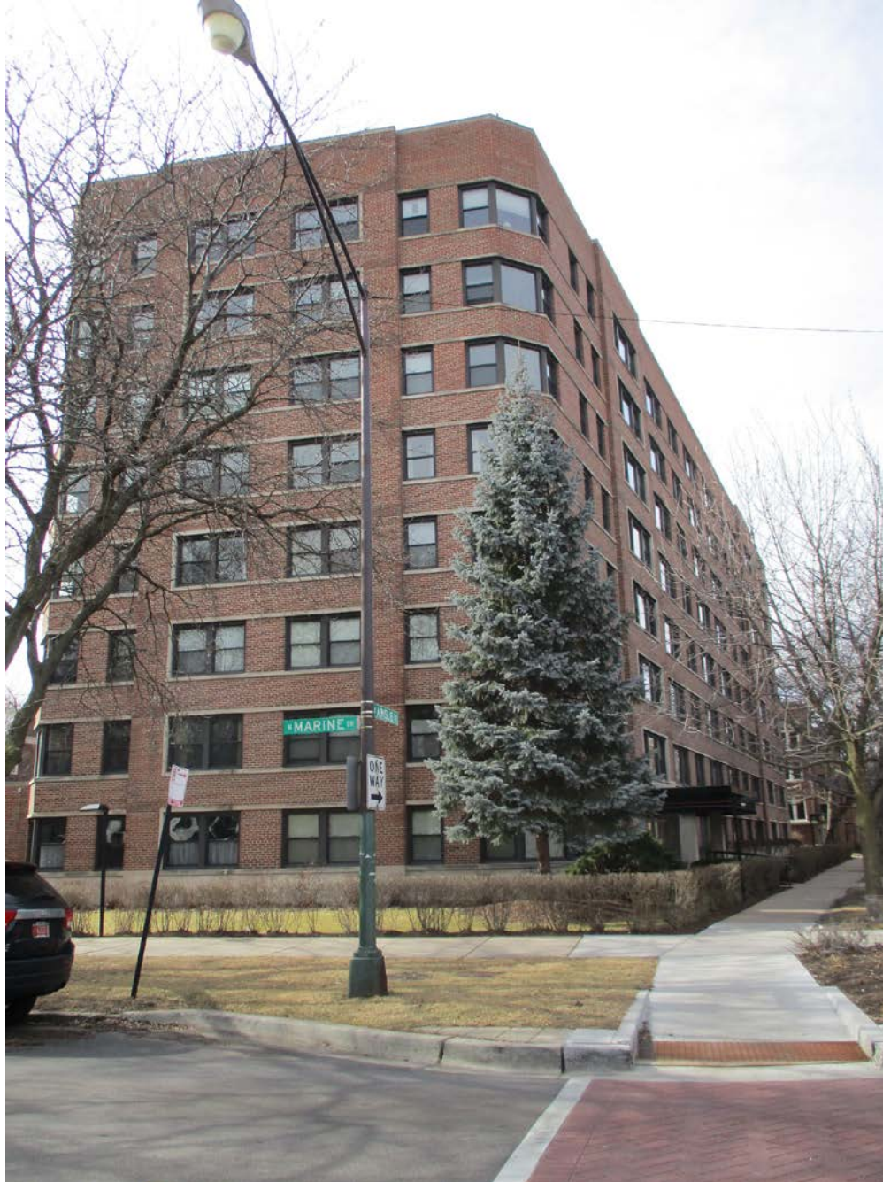
4880 N. Marine Drive, view looking west from N. Marine Drive toward East façade
