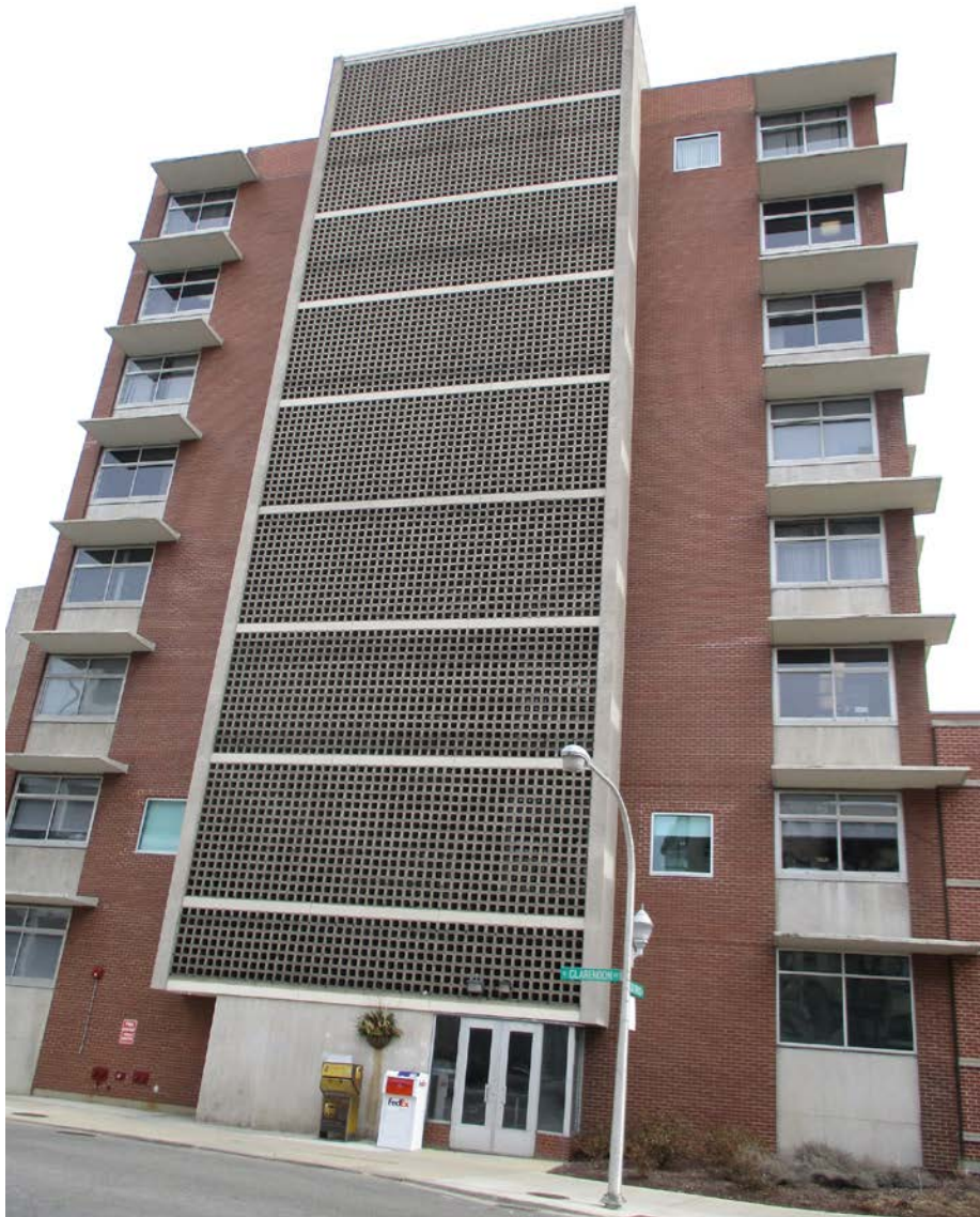
4646-4720 N. Marine Drive, view looking east from N. Clarendon Avenue toward West façade of South block
