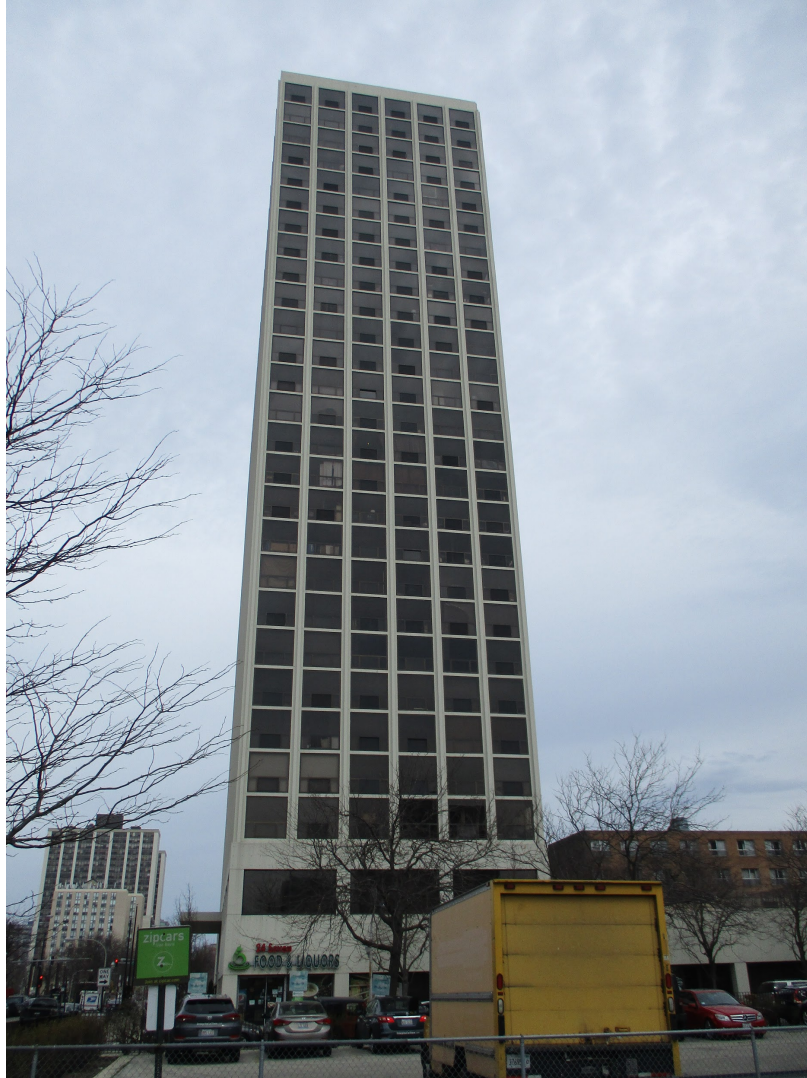
4343 N. Clarendon Avenue, view looking north from W. Junior Terrace toward South façade
