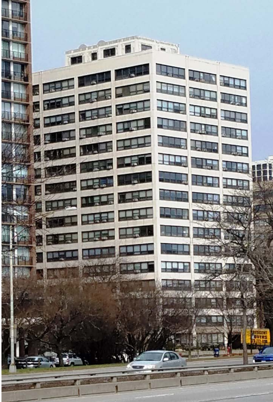
4180 N. Marine Drive, view looking northwest from N. Lake Shore Drive toward South and East façades
