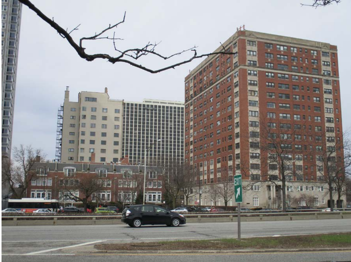
4300 N. Marine Drive (right), view looking west from N. Lake Shore Drive toward South and East façades
