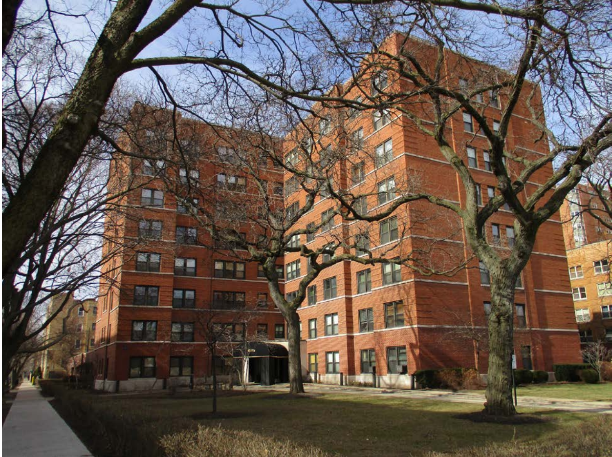
4900 N. Marine Drive, view looking southwest from N. Marine Drive toward primary entryway at Southeast building corner
