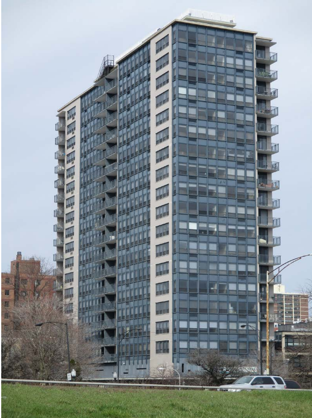
4100 N. Marine Drive, view looking northwest from N. Lake Shore Drive toward South and East façades
