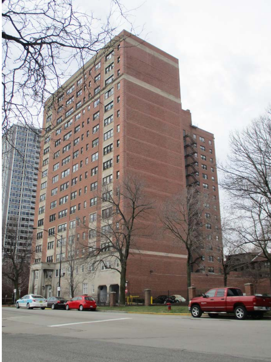
4300 N. Marine Drive, view looking southwest from N. Marine Drive toward East and North façades
