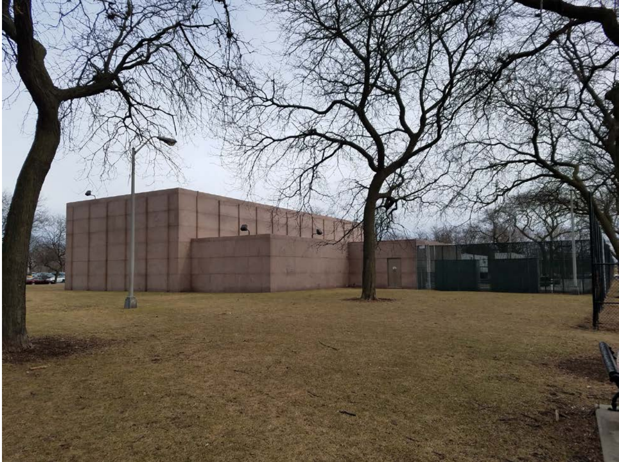
745 W. Wilson Avenue, view looking northeast from Clarendon Park toward West and South façades
