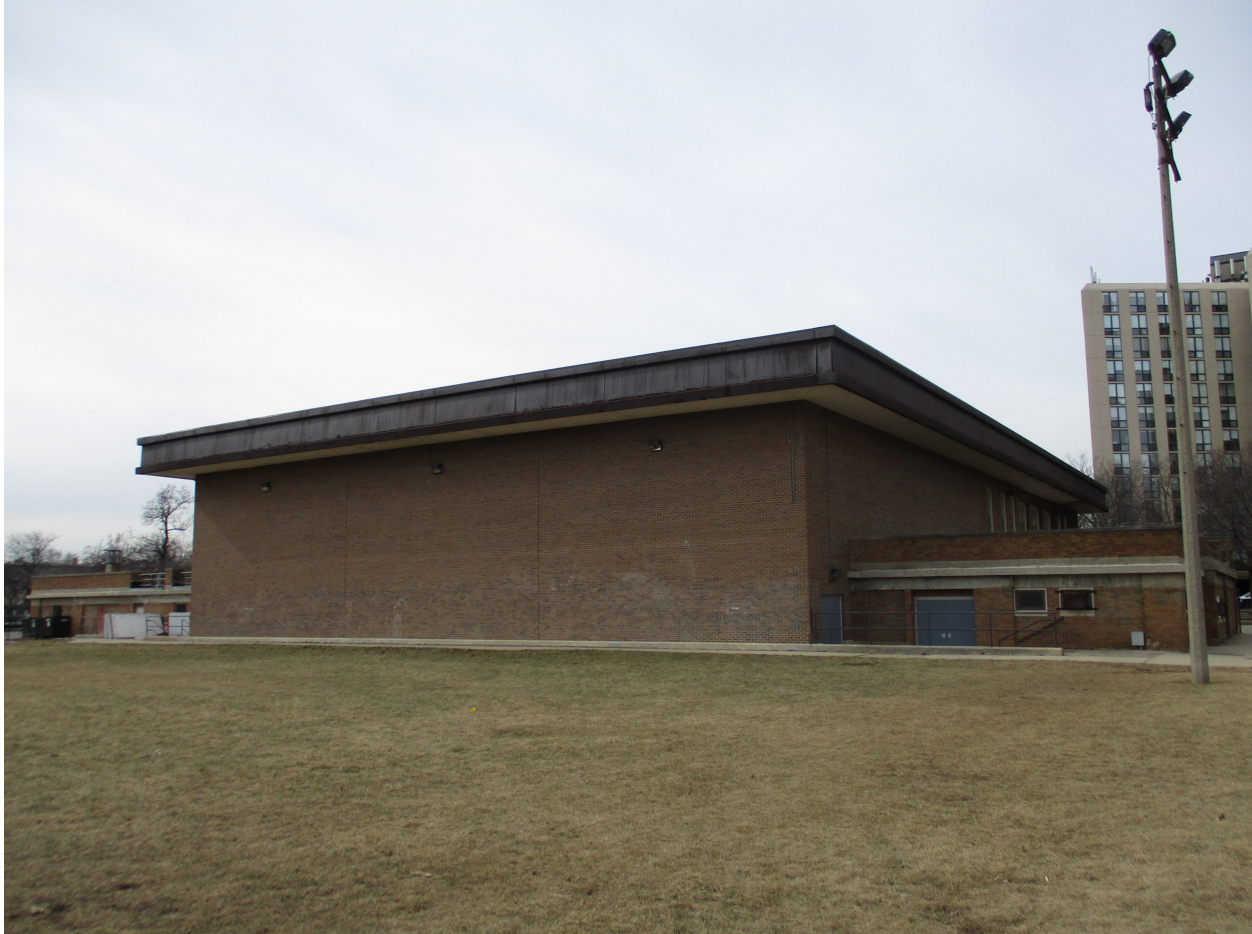
4501 N. Clarendon Avenue, view looking southwest from park toward East façade
