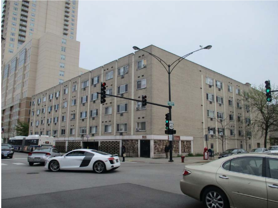
949-955 W. Foster Avenue, view looking southeast from N. Sheridan Road toward North and West façades
