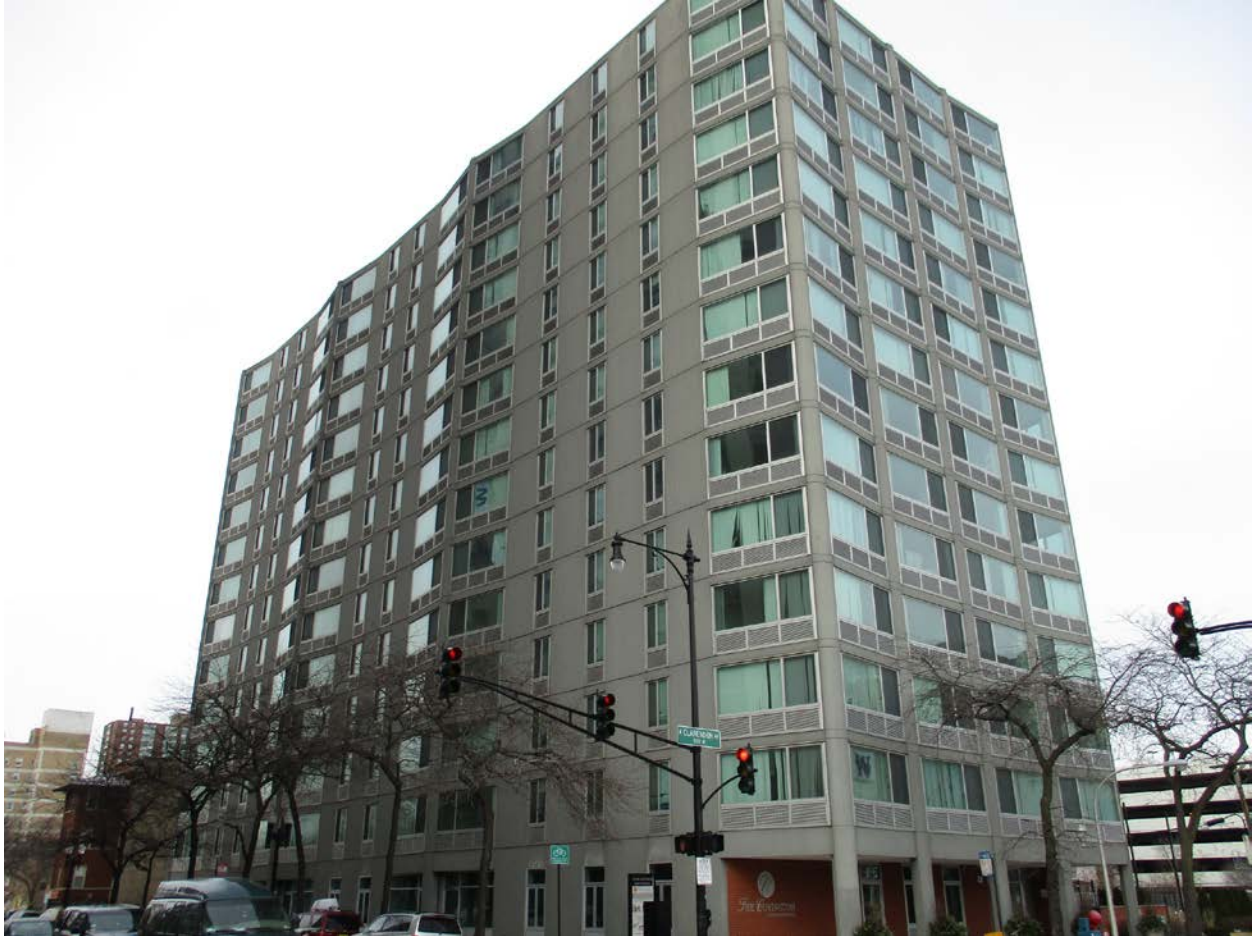
4600 N. Clarendon Avenue, view looking northwest from N. Clarendon Avenue toward South and East façades
