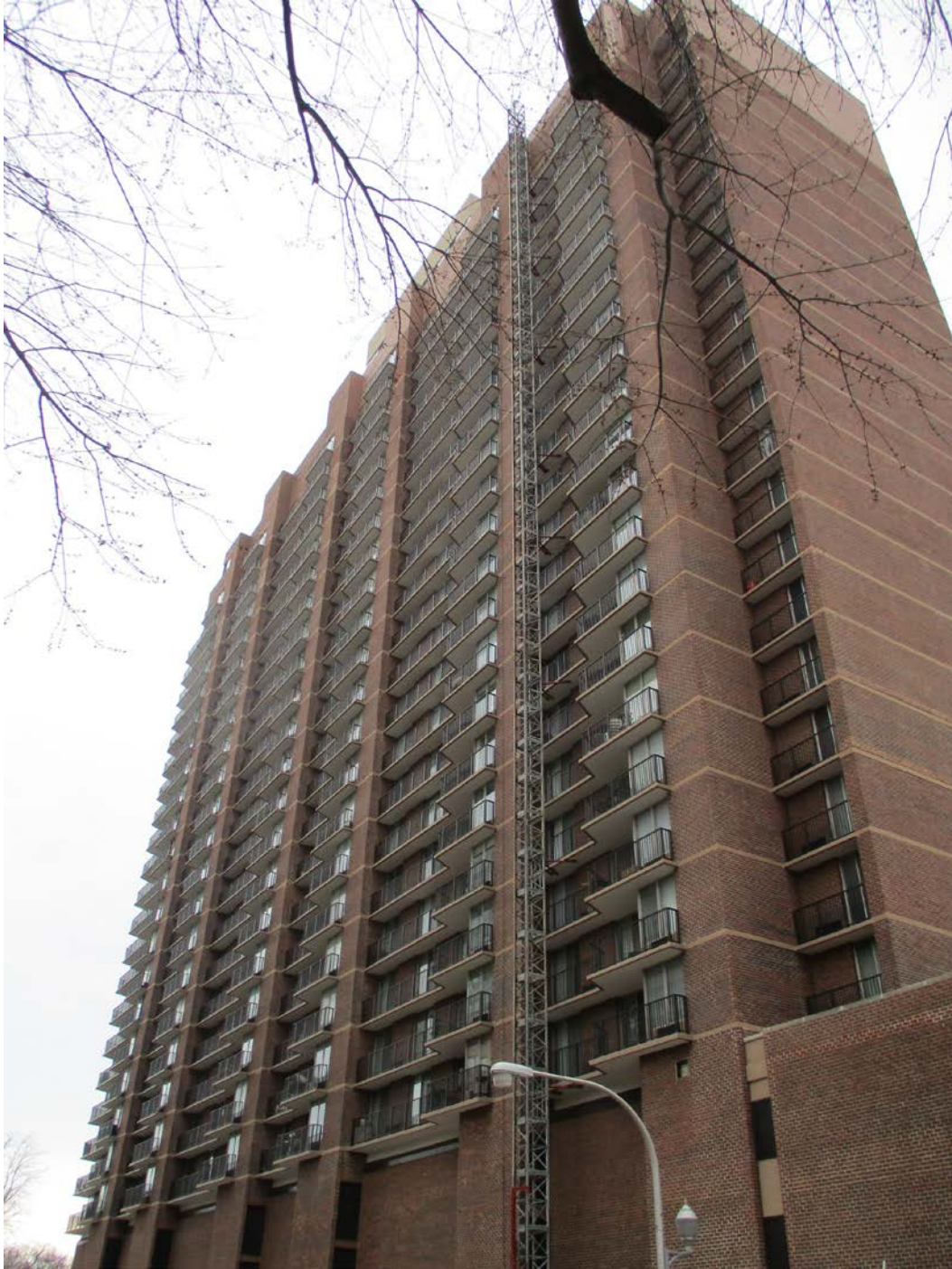
4170 N. Marine Drive, view looking southeast from W. Gordon Terrace toward North and West façades
