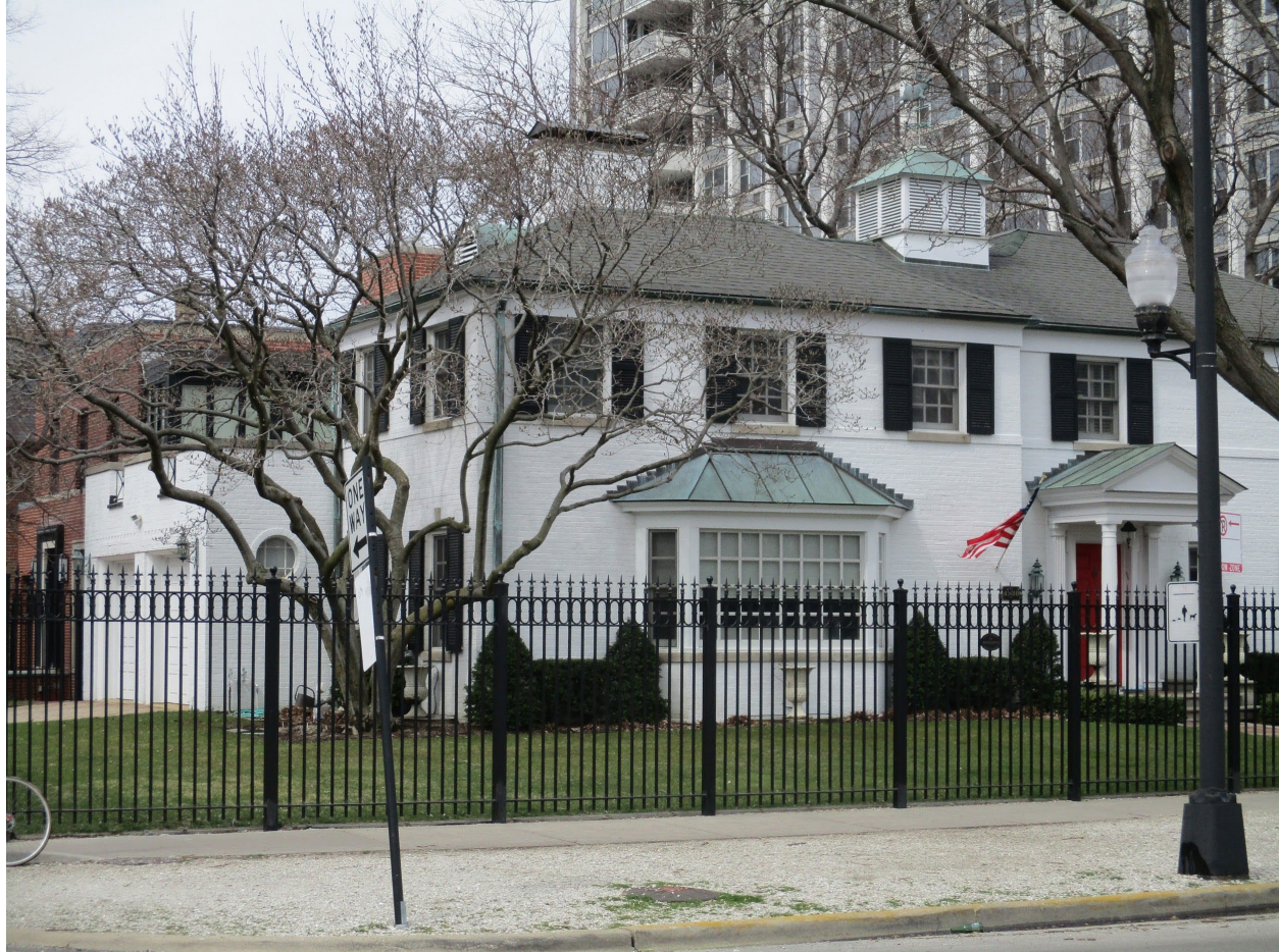
4230 N. Marine Drive, view looking northwest from N. Marine Drive toward South and East façades
