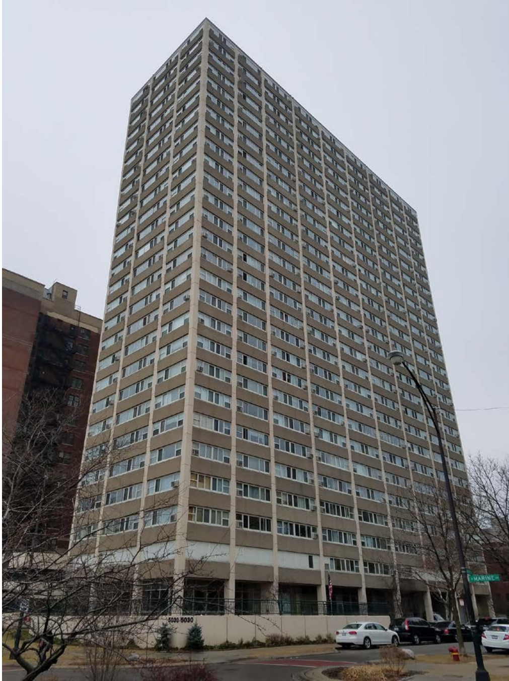
5030 N. Marine Drive, view looking southwest from N. Marine Drive toward East and North façades
