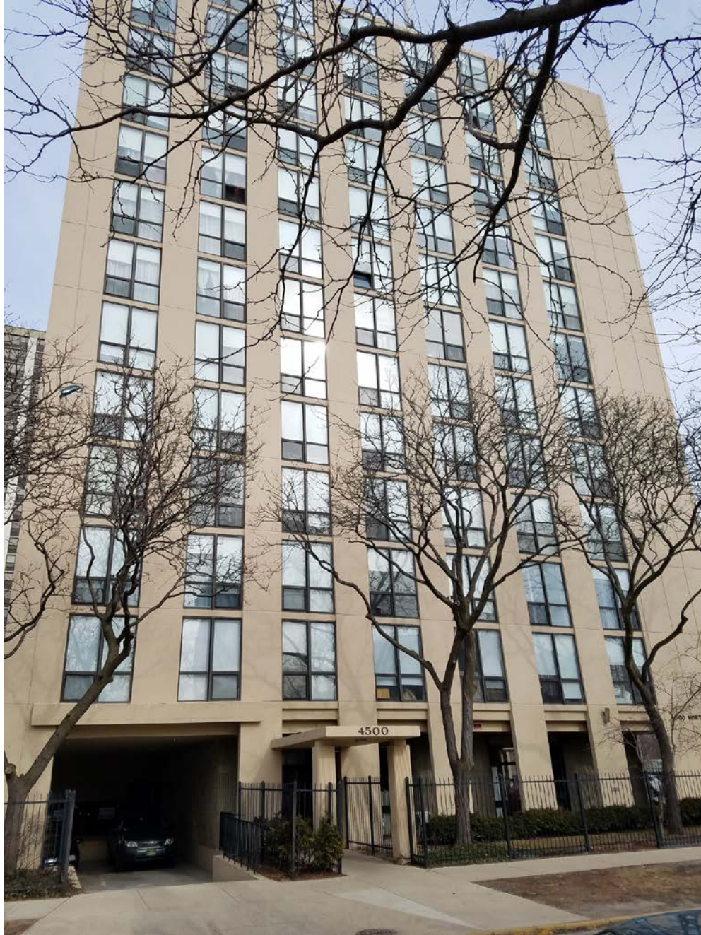
4500 N. Clarendon Avenue, view looking northeast from W. Sunnyside Avenue toward South façade
