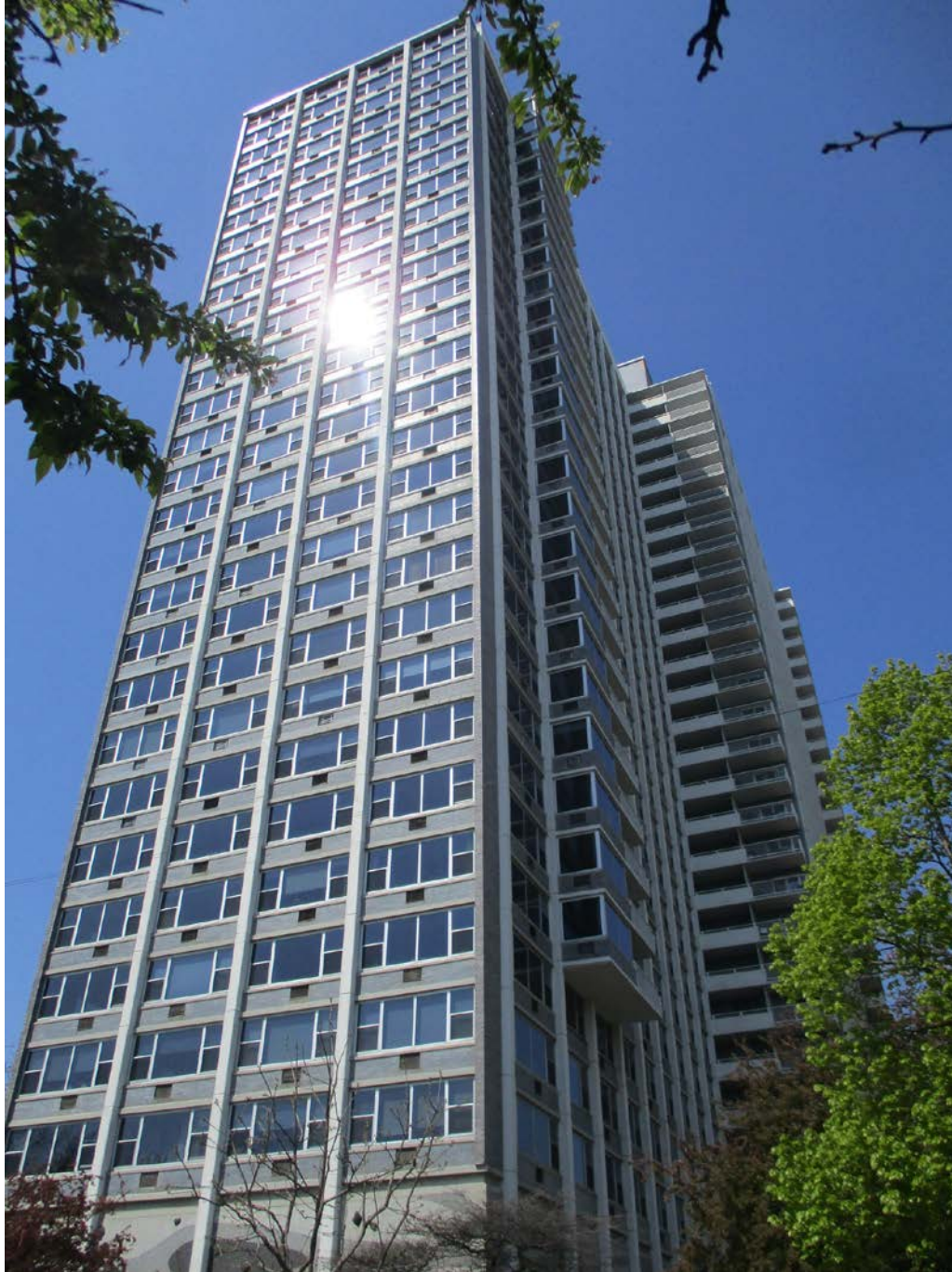
4250 N. Marine Drive, view looking southwest from N. Marine Drive toward East and North façades of South tower
