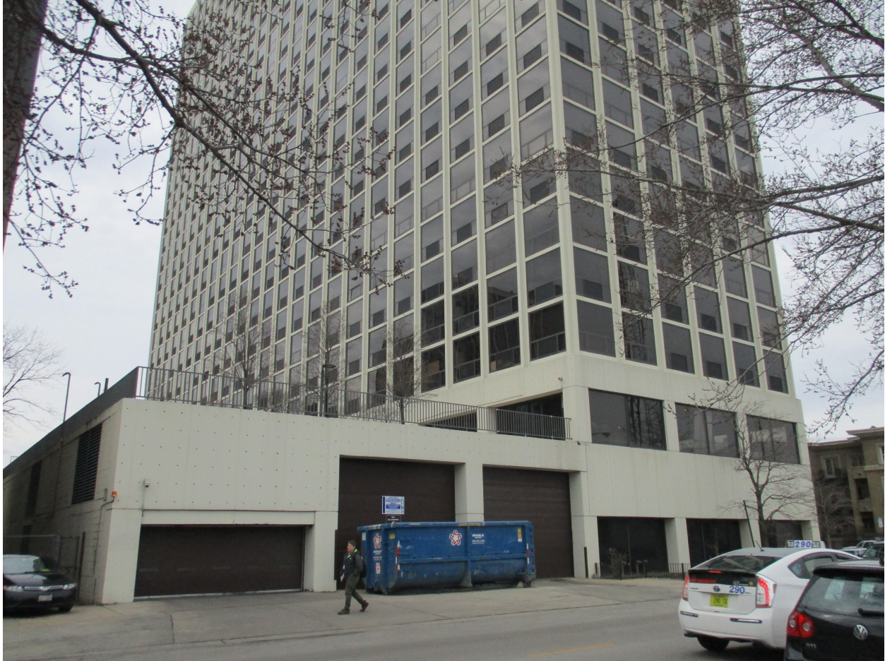
4343 N. Clarendon Avenue, view looking southwest from W. Montrose Avenue toward East and North tower façades and East terrace wing
