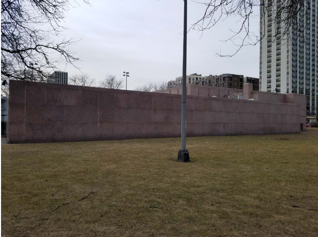
745 W. Wilson Avenue, view looking southwest from Clarendon Park toward North façade
