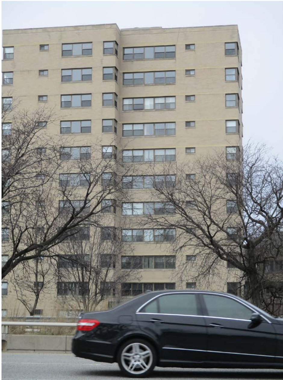
4200 N. Marine Drive, view looking west from N. Lake Shore Drive toward East façade
