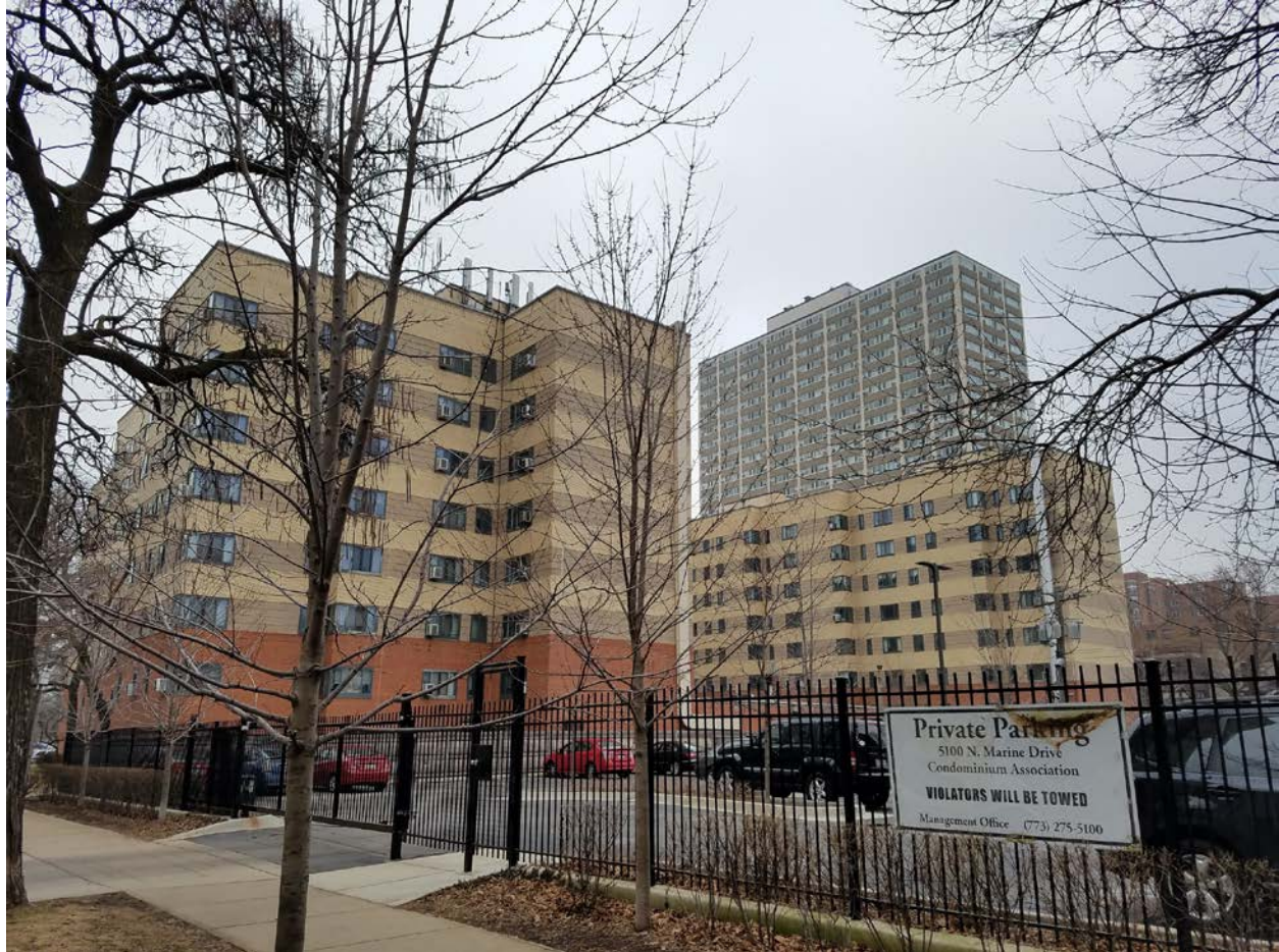
5040-5060 N. Marine Drive looking southeast from W. Winona St. toward the West facade.
