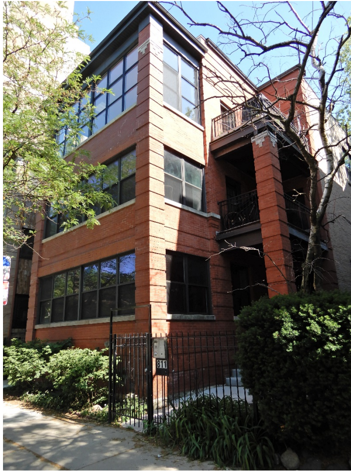
811 W. Lawrence Avenue, view looking southeast from W. Lawrence Avenue toward north and west façades
