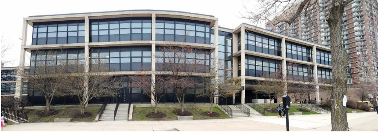
4140 N. Marine Drive, panorama view looking northwest from N. Marine Drive toward East façade
