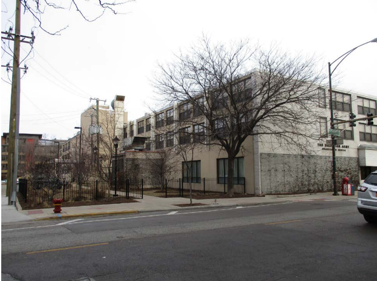
800 W. Lawrence Avenue looking northeast from W. Lawrence Avenue toward West and South facades.
