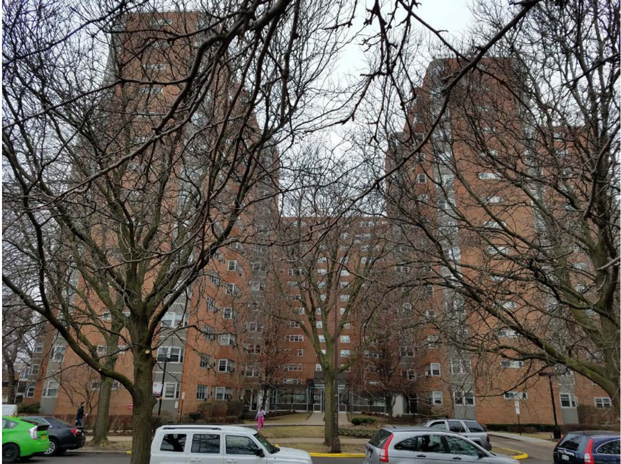
4950-4980 N. Marine Drive, view looking west from N. Marine Drive toward primary East façade and courtyard
