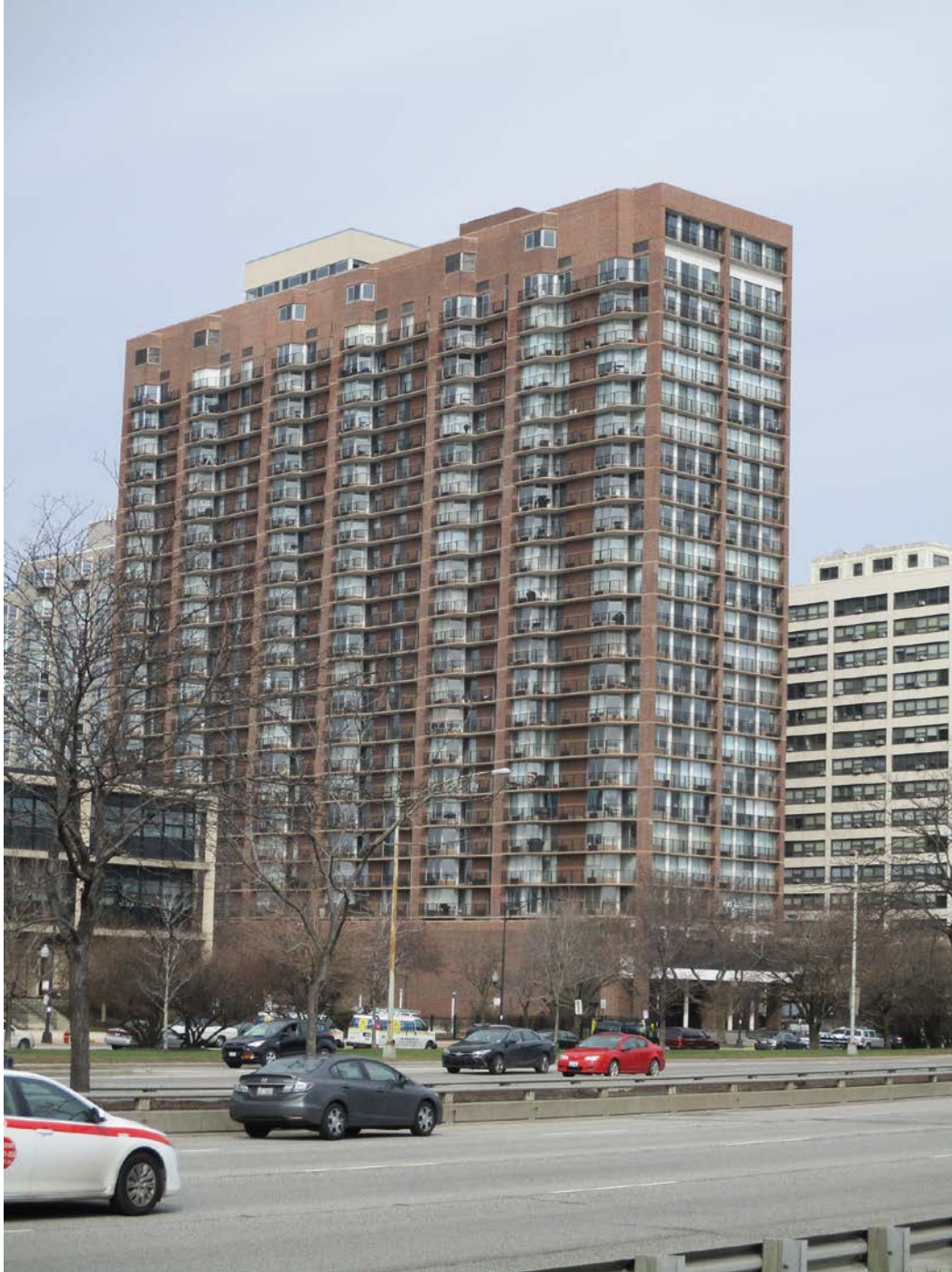
4170 N. Marine Drive, view looking northwest from N. Lake Shore Drive toward South and East façades
