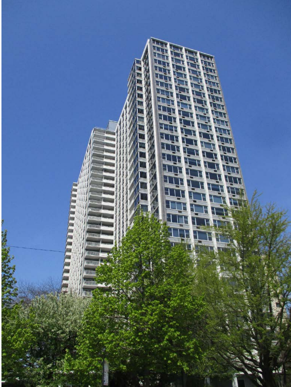
4250 N. Marine Drive, view looking northwest from N. Marine Drive toward South and East façades of North Tower
