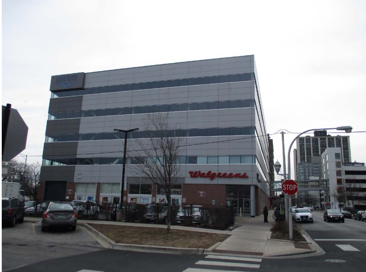
4646-4720 N. Marine Drive, view looking south from W. Lakeside Place toward North façade of Lakeshore Medical Center (2008 addition)
