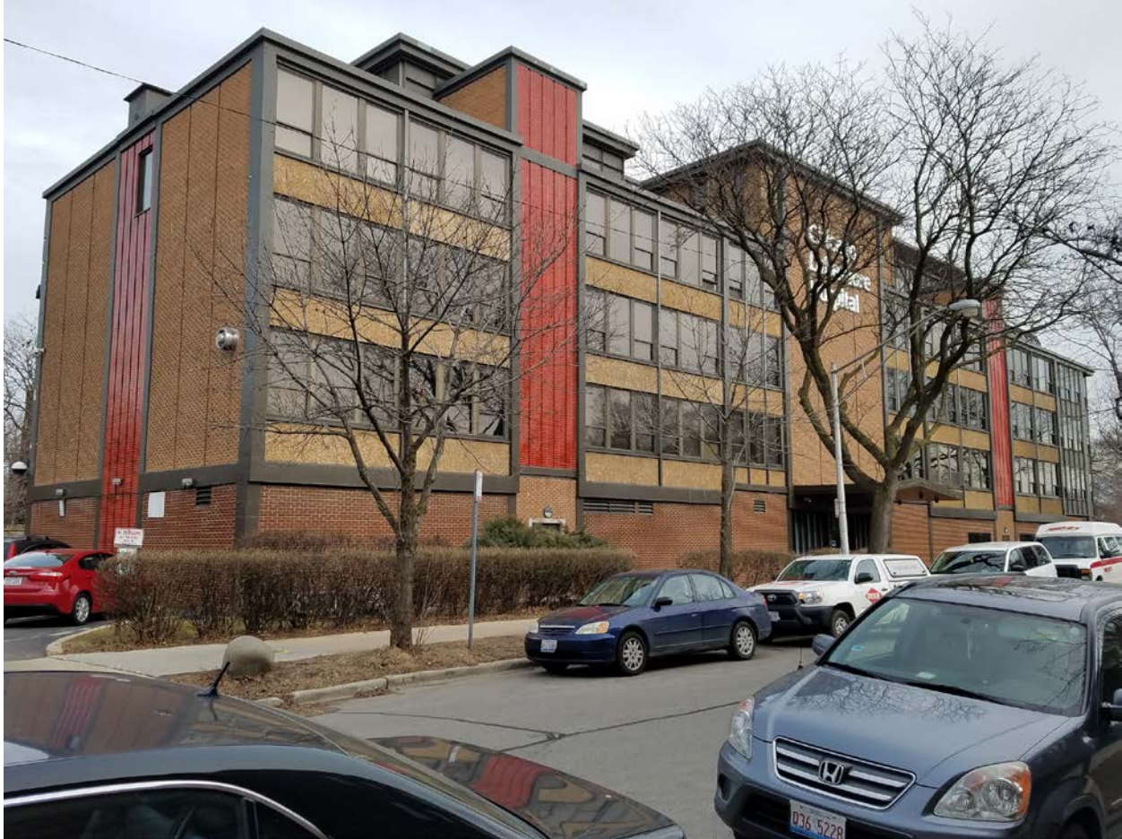
4840 N. Marine Drive, view looking northeast from W. Gunnison Street toward West and primary South façades
