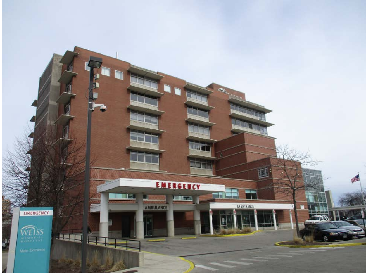
4646-4720 N. Marine Drive, view looking northeast from parking lot toward South façade of South block
