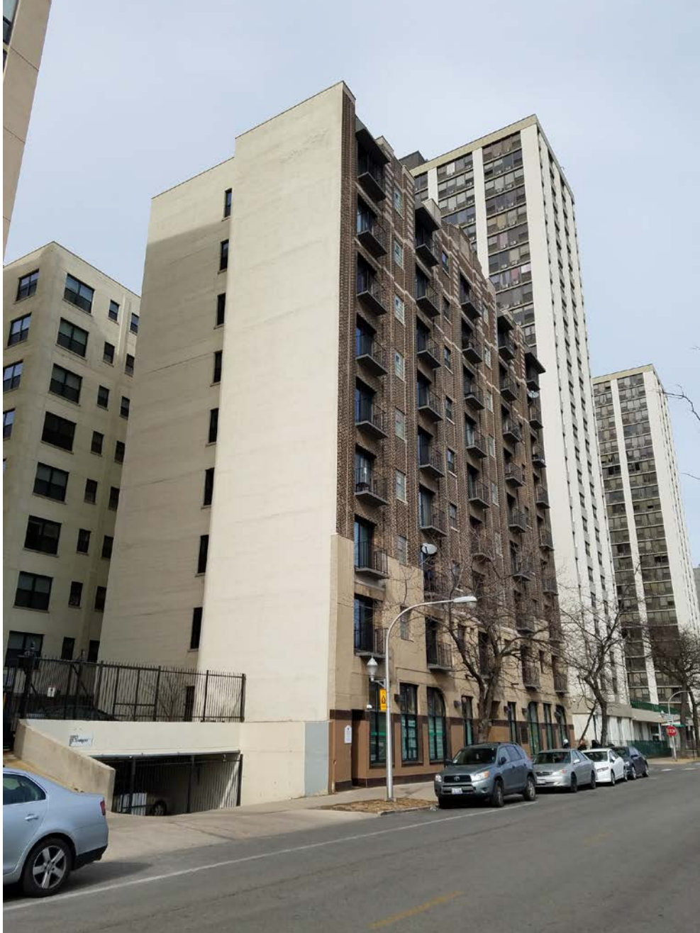
4520 N. Clarendon Avenue, view looking northwest from N. Clarendon Avenue toward East and South facades
