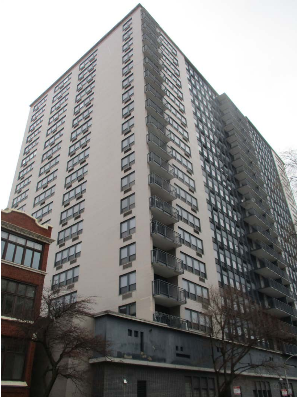
4100 N. Marine Drive, view looking northeast from W. Bittersweet Place toward West and South façades
