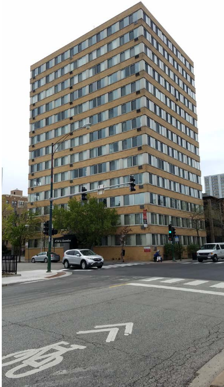
4750 N. Clarendon Avenue, view looking southwest from W. Lawrence Avenue toward East and North façades
