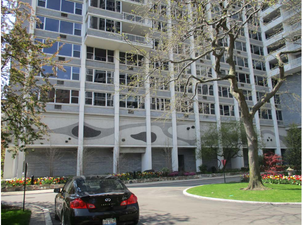
4250 N. Marine Drive, view looking southwest from driveway toward base-level detail on North façade of South tower
