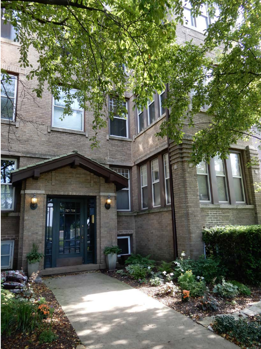
717-719 W. Montrose Ave., view looking southeast toward main entrance of North facade
