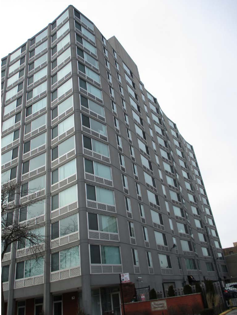
4600 N. Clarendon Avenue, view looking southwest from N. Clarendon Avenue toward North façade
