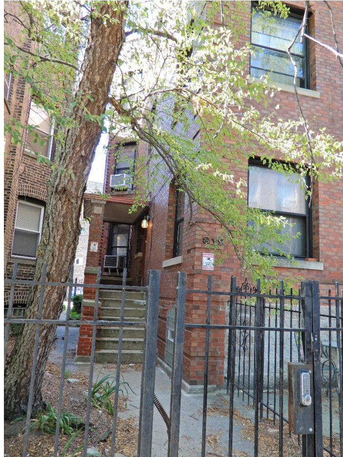
819 W. Lawrence Avenue, view looking south from W. Lawrence Avenue toward entryway
