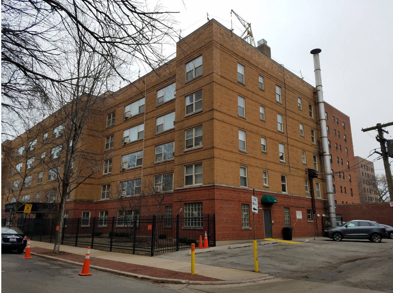
4920 N. Marine Drive, view looking southeast from W. Margate Terrace toward West façade
