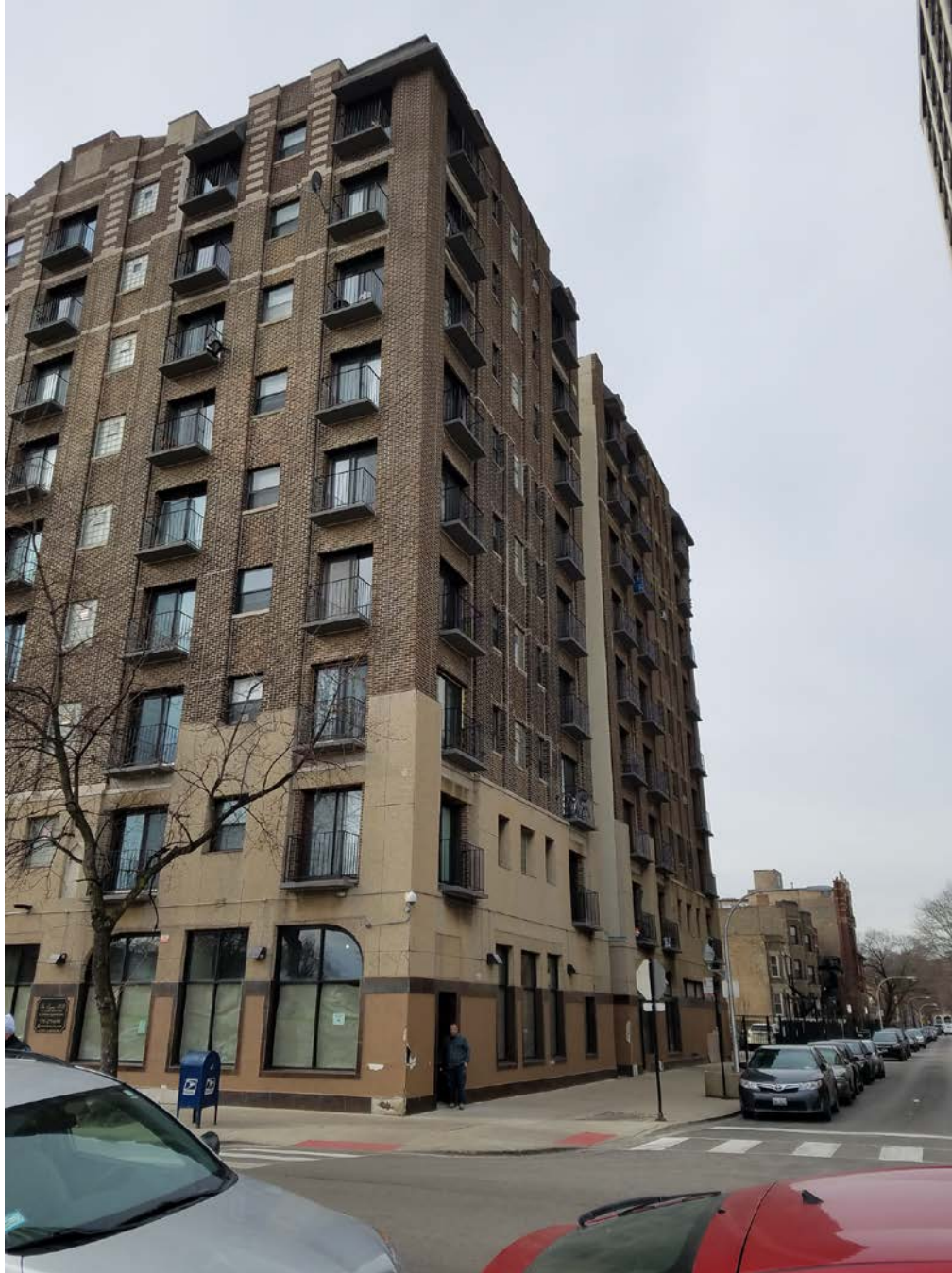
4520 N. Clarendon Avenue, view looking southwest from N. Clarendon Avenue toward East and North facades
