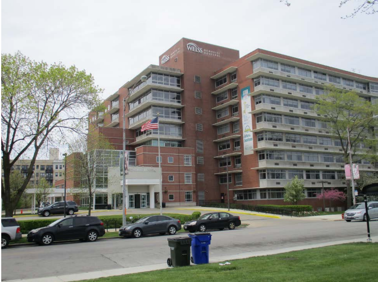
4646-4720 N. Marine Drive, view looking northwest from N. Marine Drive toward the intersection of the South block (left) and original East-facing 1953 building (right)
