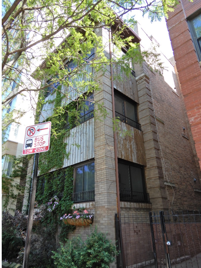
809 W. Lawrence Avenue, view looking southeast from W. Lawrence Avenue toward north and west façade
