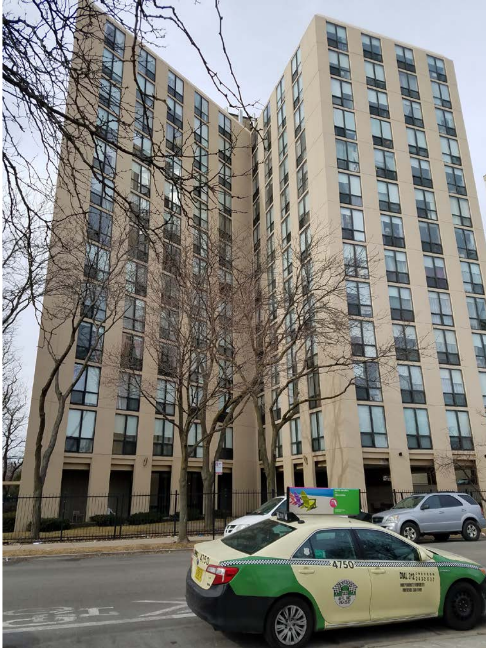
4500 N. Clarendon Avenue, view looking northwest from N. Clarendon Avenue toward East façade
