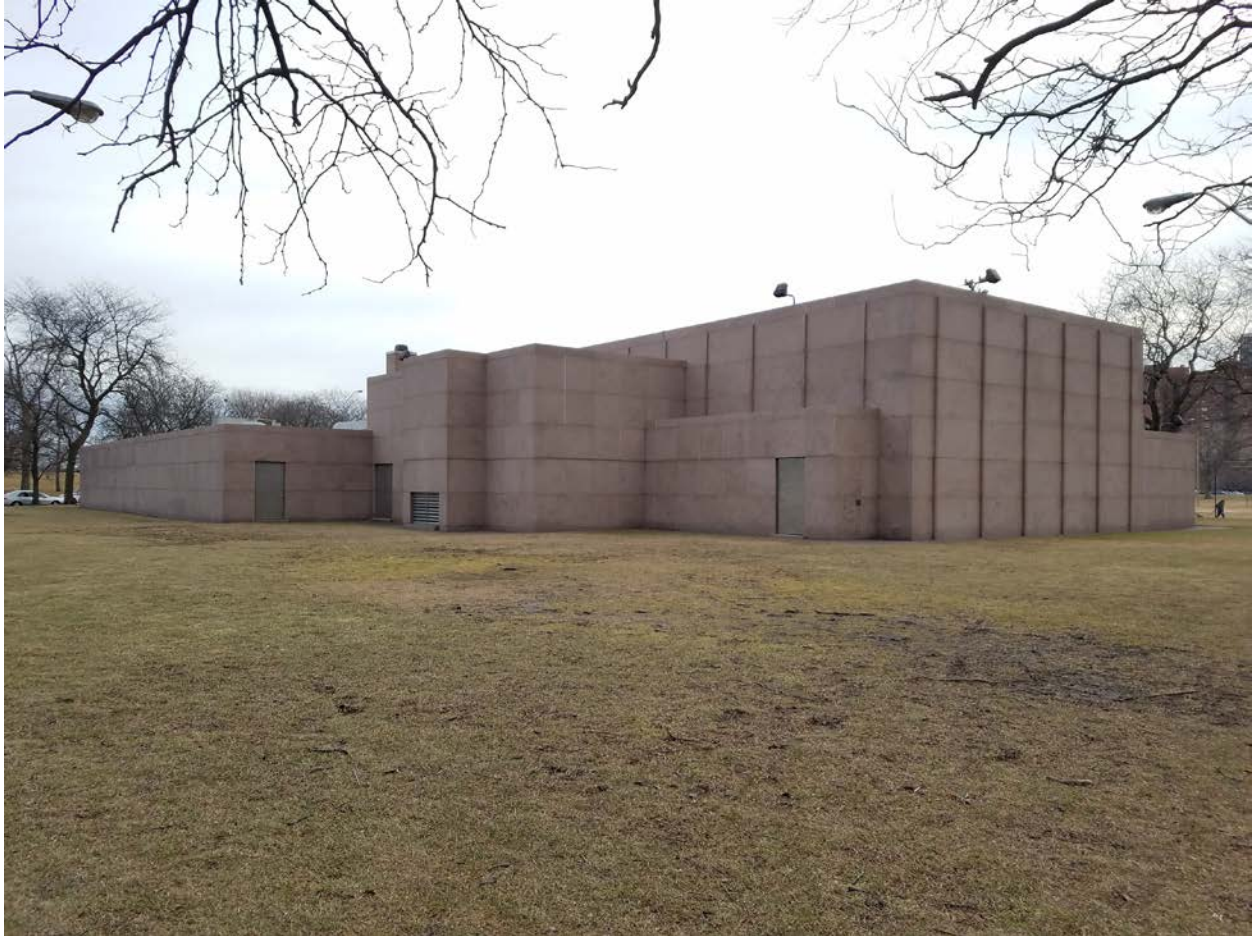
745 W. Wilson Avenue, view looking southeast from Clarendon Park toward North and West façades
