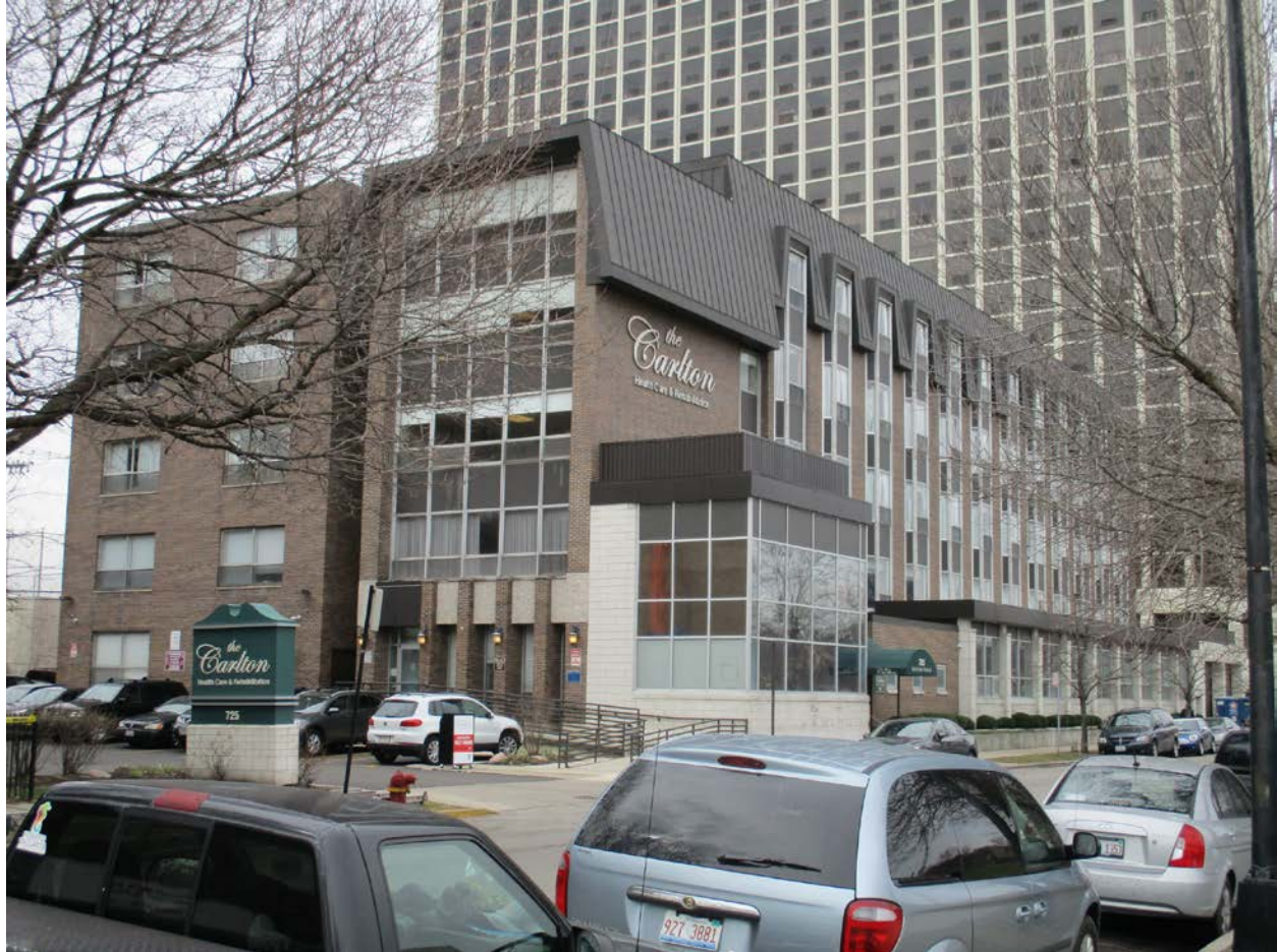
725 W. Montrose Avenue, view looking southwest from W. Montrose Avenue toward East façade
