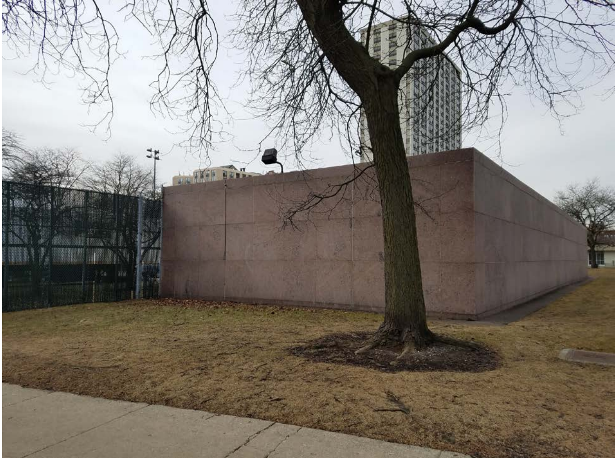
745 W. Wilson Avenue, view looking west from N. Marine Drive toward East façade
